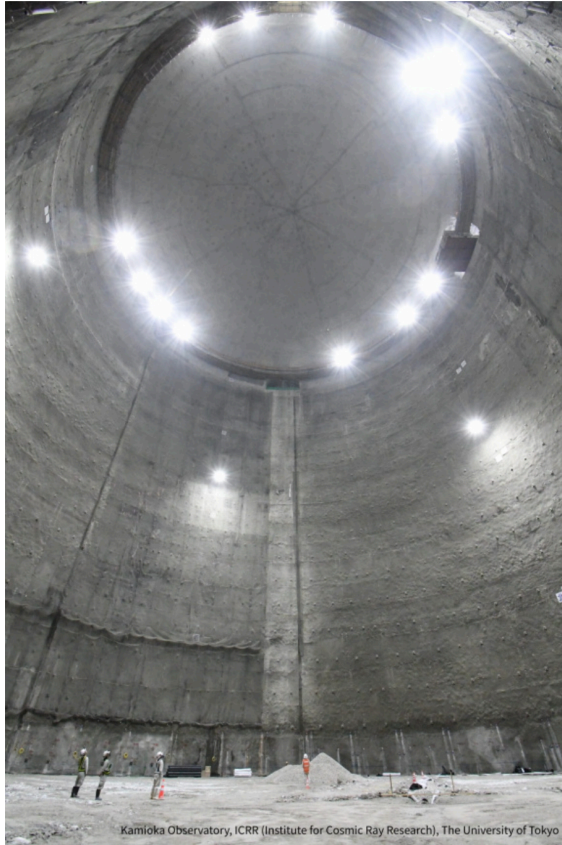
The main Hyper-Kamiokande cavern after excavation completed
