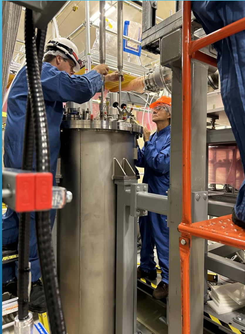
50K Cooler installation
