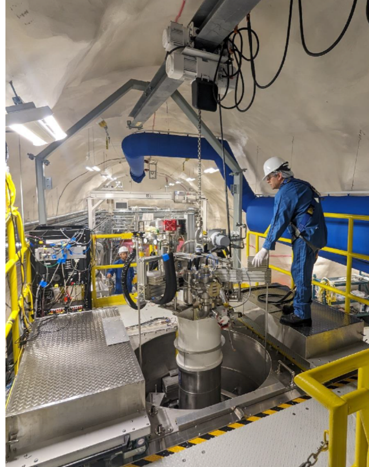
Lowering of DR into drywell
